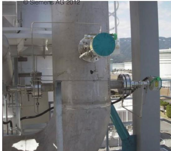
Pointek CLS level switch for overspill protection or interface detection
