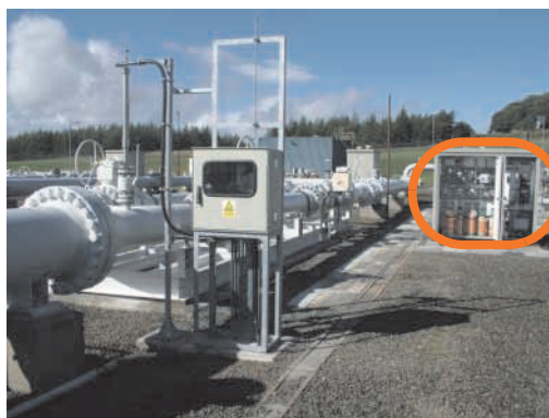
Fig. 7: SITRANS CV installation in a metering station
