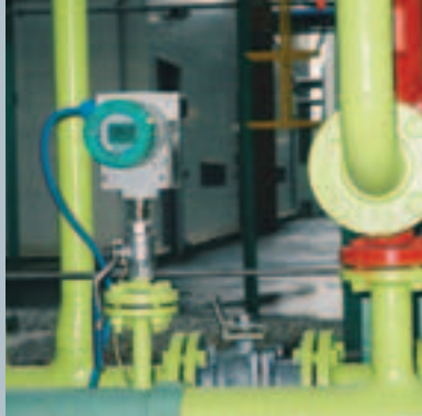
Absolute pressure measurement with SITRANS P in a loading system for toluene
