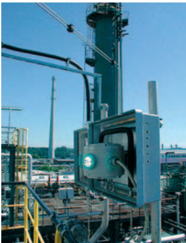
Direct oxygen and ethylene measuring at an EDC (ethylene di-chloride) boiling reactor with a process gas chromatograph
