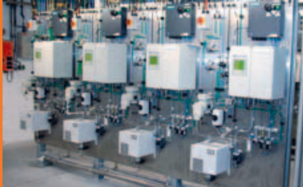
Analysis house with process gas analyzers and sample preparation in an acrylic acid plant
