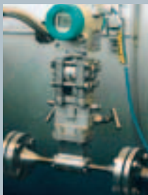
Flow measurement at a measuring orifice with SITRANS P
