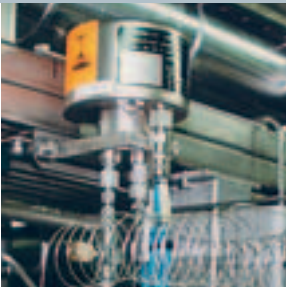
Often used in pilot systems or for dosing applications: Coriolis flowmeter SITRANS FC for small flowrates
