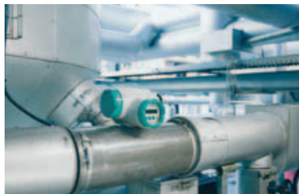
Ultrasound flowmeter SITRANS F US in a formaldehyde production plant
