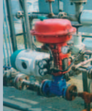
SIPART PS2 positioner with explosion protection in a chemical plant
