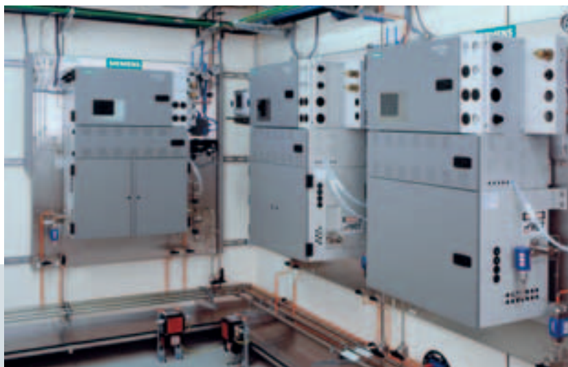
Process gas chromatograph in the analysis house of an aromatics plant
