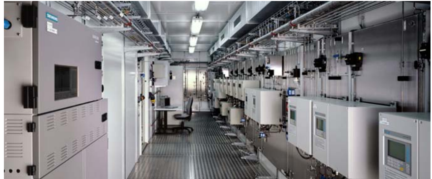
Fig. 20: Analyzer shelter
