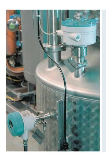
Tried and tested for a wide range of applications, Siemens inverse frequency shift capacitance continuous level transmitters are suitable for liquids, solids, and interface applications. Siemens capacitance instruments use active-shield technology to ensure true and accurate level readings are recorded from the material surface.
