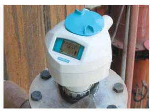
The SITRANS LR250 with SIL 2, in accordance with the IEC 61508/61511 standard for Functional Safety, features longer confirmation cycles than those of its competition, as well as a higher Safe Failure Fraction (SFF), both distinct benefits to customers.
