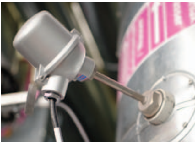
Monitoring temperatures with SITRANS T to boost efficiency in the Kalina process
