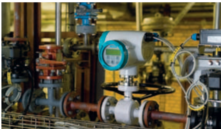
Electromagnetic flowmetering in an explosion hazard area with the SITRANS FM
