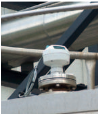
Storage tank level measurement with SITRANS LR
