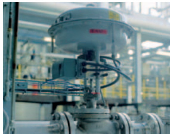
SIPART PS2 – the most frequently used intelligent positioner for linear and rotary actuators
