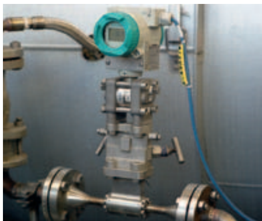
Flow measurement at a measuring orifice with SITRANS P
