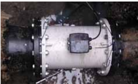
Distribution and abstraction: MAG 8000 minimizes maintenance and detects leaks early
