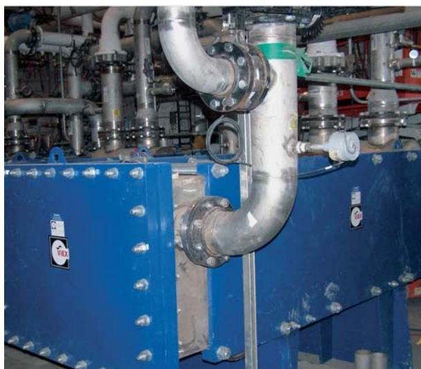
Temperature measurement with SITRANS T on a mash cooler
