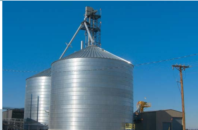
Storage tanks for corn. In each silo, a SITRANS LR 400 measures the actual level in the hazardous dust area
