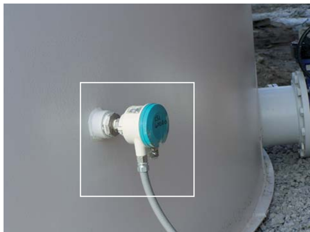
Monitoring of minimum level on a tank using POINTEK
