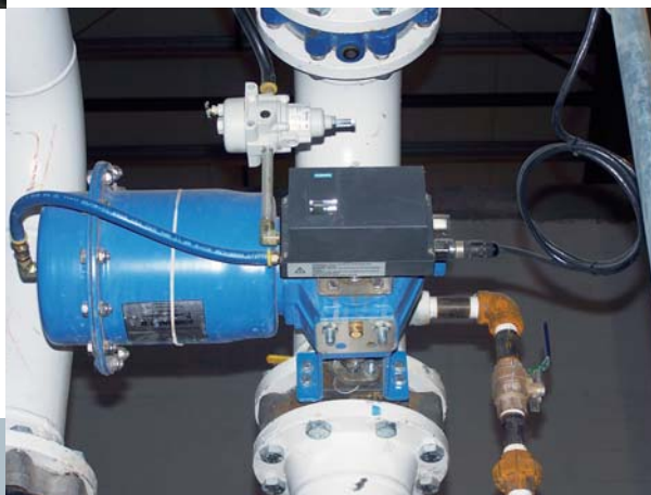
Valve control with SIPART PS2 in a continuous fermentation plant
